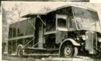
B.B.C. mobile television transmitter—the two photos—above and at the right—show the powerful mobile television unit which can be dispatched to cover news events anywhere on short notice. The truck has a television transmitter and can relay the image and sound to a pick-up station at a considerable distance; or if a television cable of the coaxial type is at hand, the truck unit can be plugged into the cable, which then carries the image and voice to the television station.
